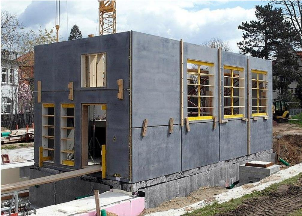
Figure 47: Construction site of Henn's Cube will, the world's first building made of carbon fiber-reinforced concrete. Taken from [Wikimedia Common](#), [CC BY-SA 4.0](#) license
